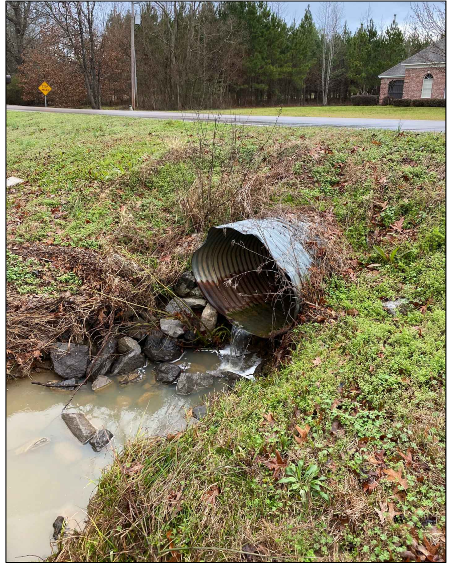
PHOTO 6: 27"x43" CMP Culvert Under Germantown Road
