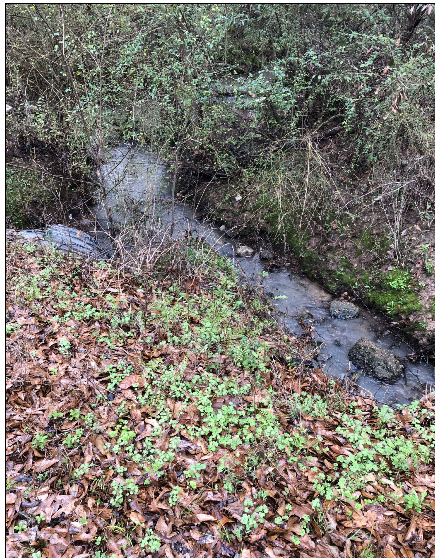
PHOTO 14: E Invert of Dbl. Culvert Under Church Road (54"x60" & 48")
