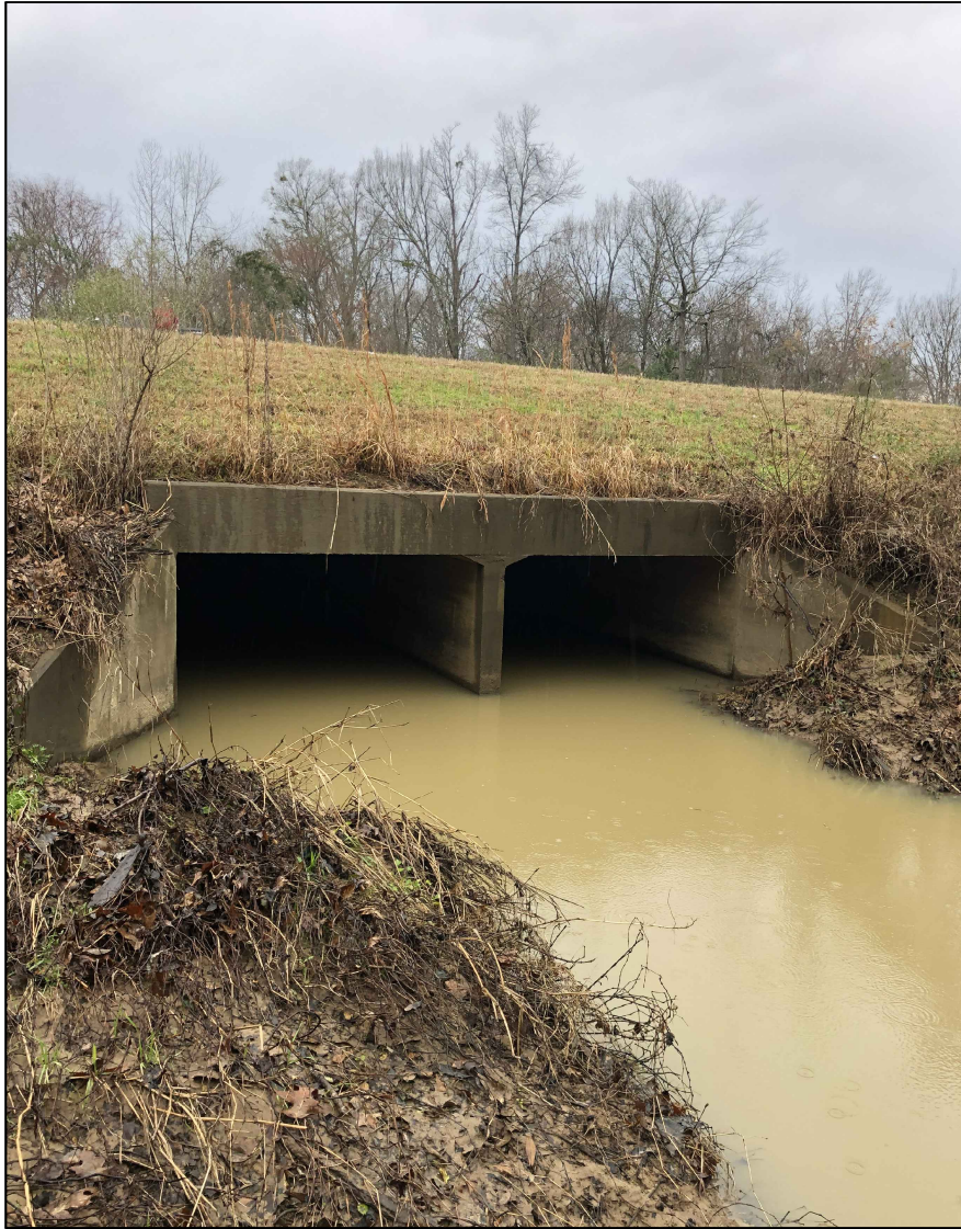
PHOTO 17: Eastern Invert of 5' x 8' Dbl Box Culvert under CSP
