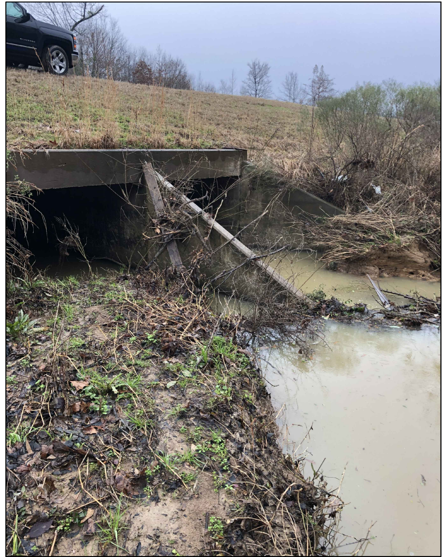
PHOTO 16: Western Invert of 5' x 8' Dbl Box Culvert under CSP
