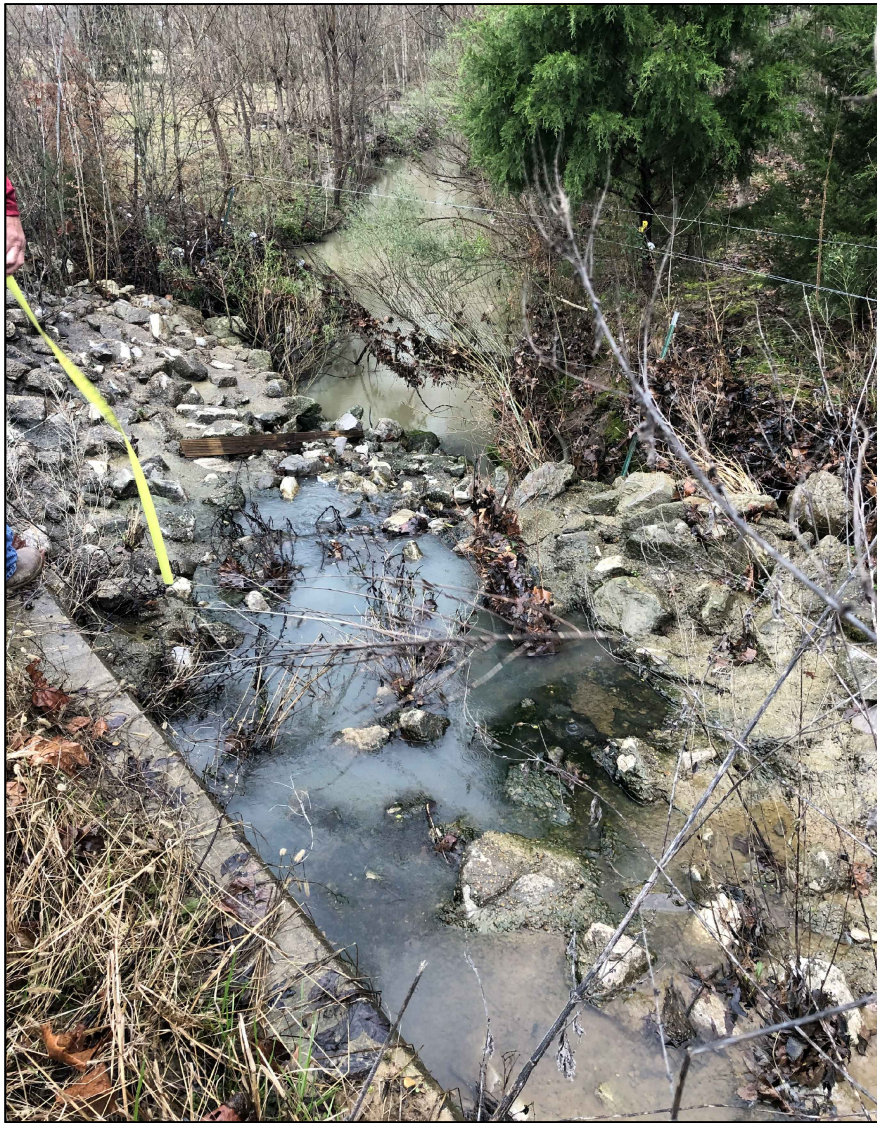
PHOTO 9: 8' x 4' Double Box Culvert Under Stribling Road
