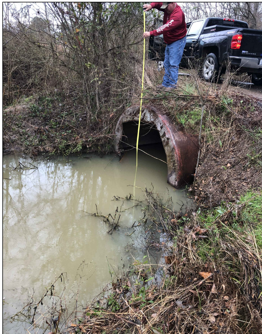
PHOTO 11: Fuel Tank X'ing at Sam Bouldin Road w/60" Opening
