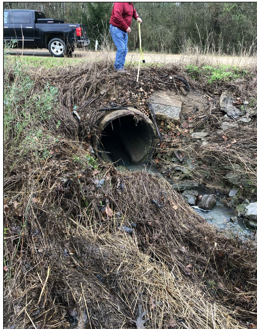
PHOTO 12: 54" Concrete Culvert Under Samuels Drive
