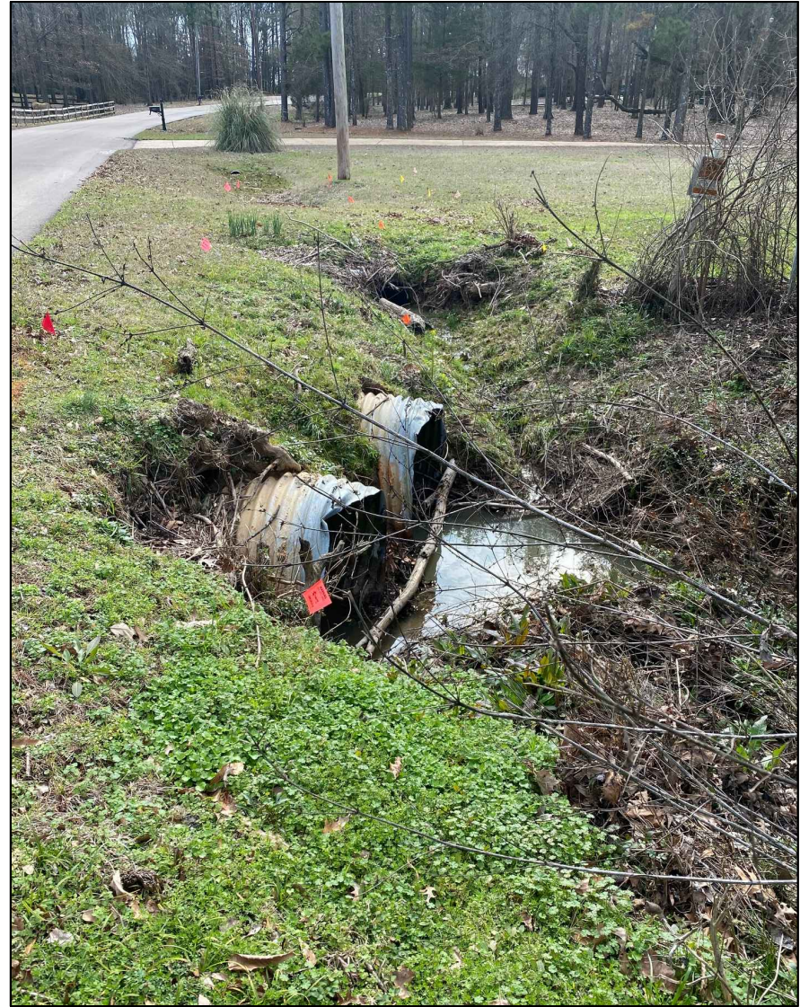
PHOTO 4: Ditch at Munich Cove, Upstream End
