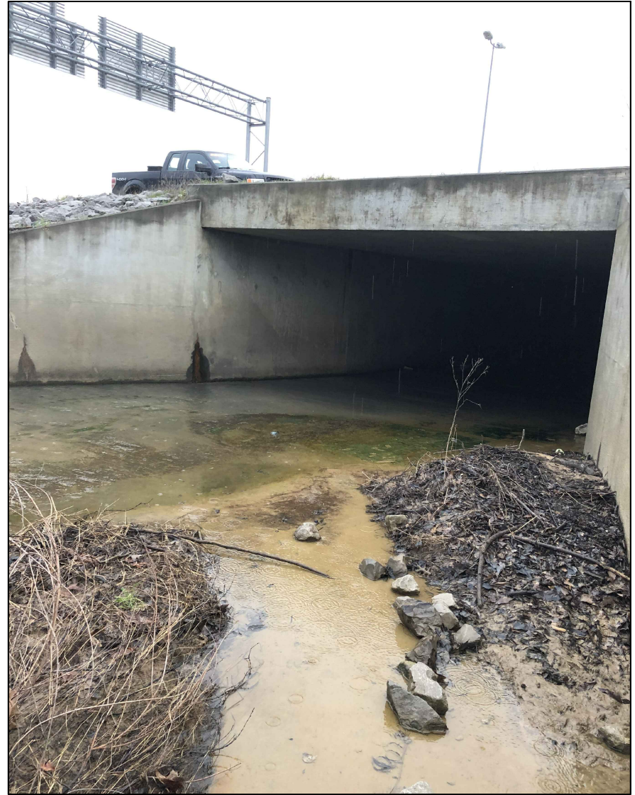
PHOTO 18: Western Invert of 20' x 8' Box Culvert under I-55
