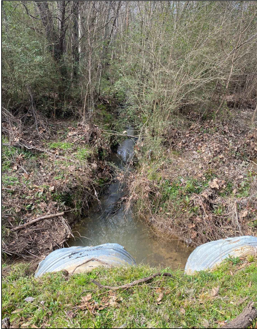
PHOTO 5: Ditch at Munich Cove Look South
