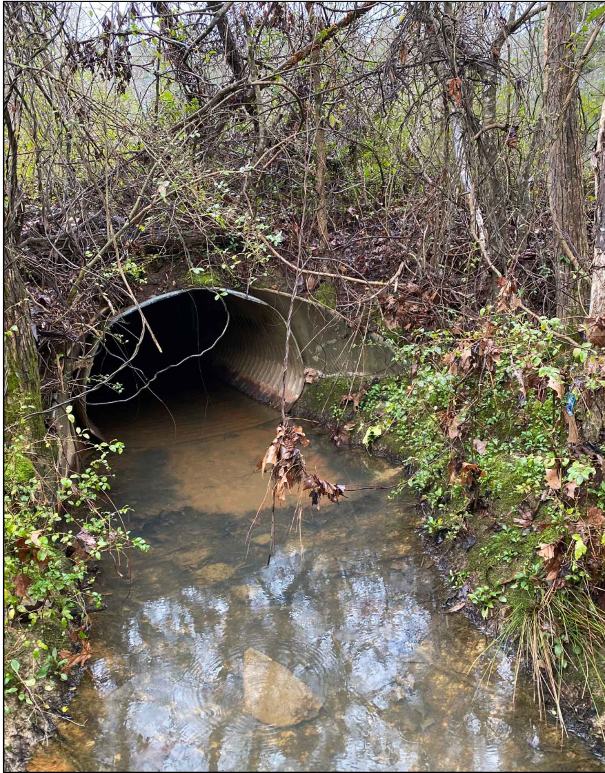
PHOTO 3: 31"x50" Culvert Under Germantown Lane
