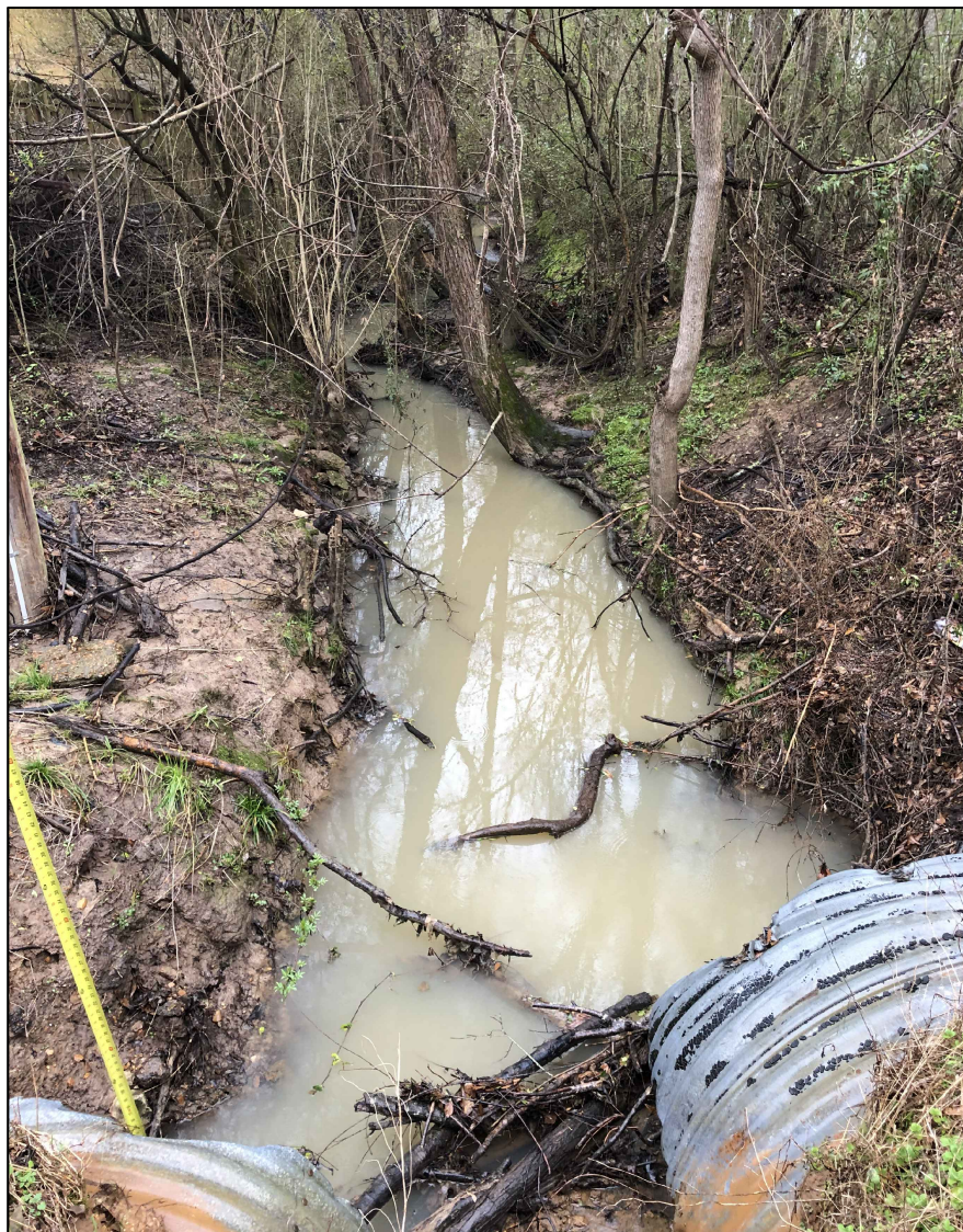
PHOTO 13: W Invert of Dbl. Culvert Under Church Road (54"x60" & 48")
